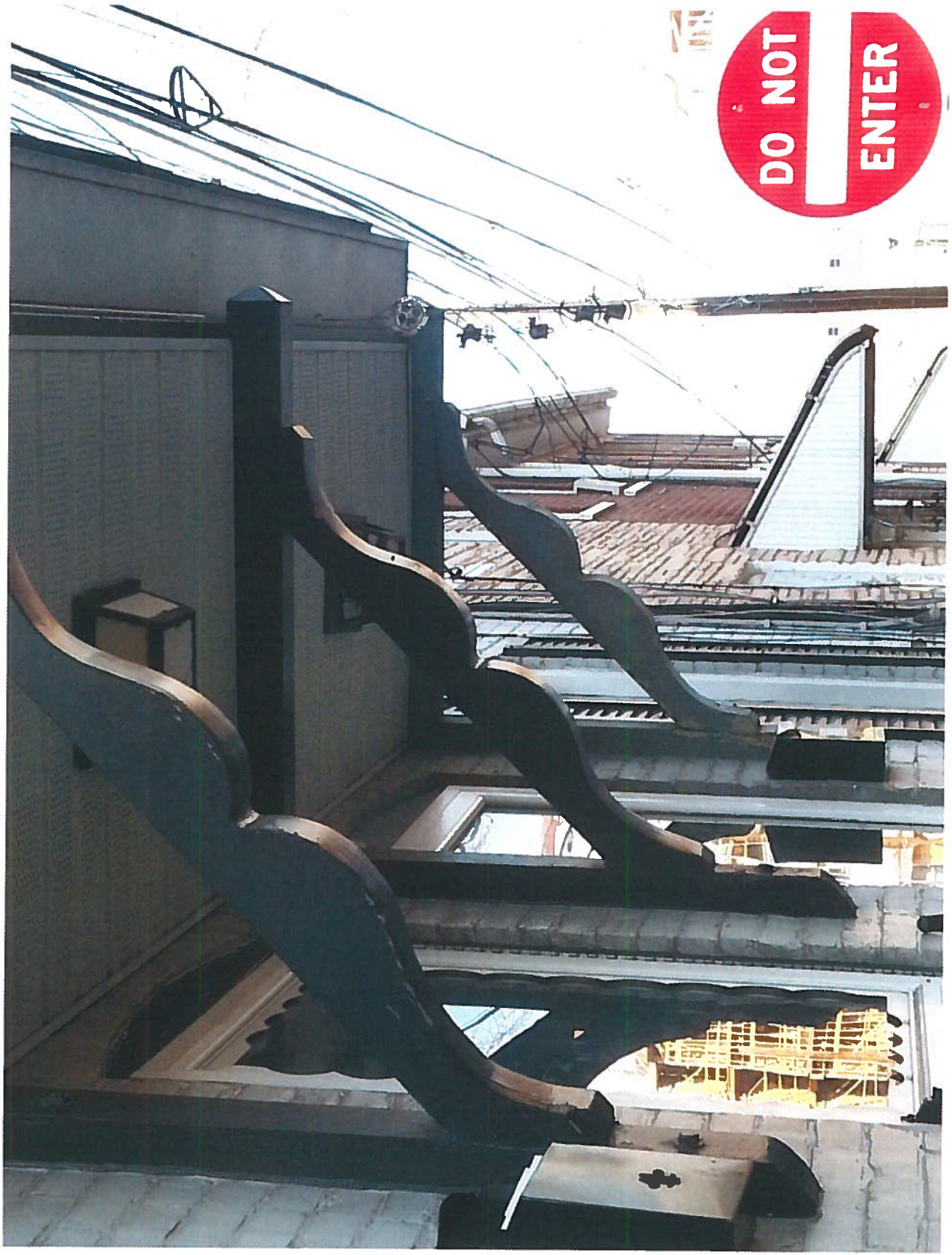
Entry Overhang Structure- side view
